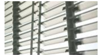
Figure 14: Detail of the stud with the twisting fins connected to it
