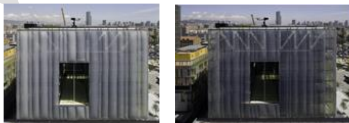
Figure 17: The opaque state when filled with nitrogen (left) and the transparent state (right) of the Southwest façade.
